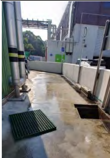
Figure.4 Completed cleanup of tank farm and nearby surface channels
