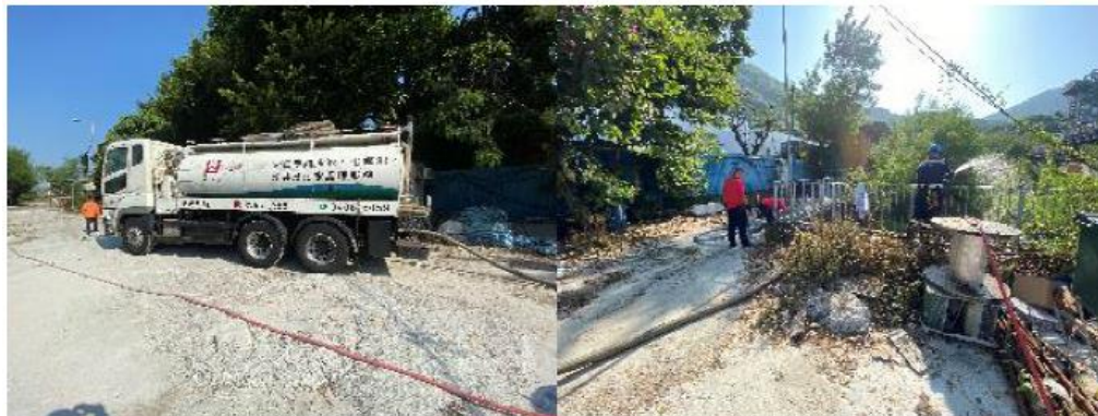
Figure.1 Vacuum tanker was arranged to cleanup the nullah
