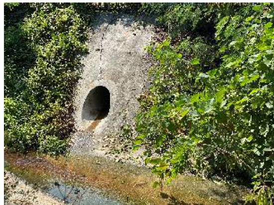
Figure.3 Complete cleanup of nullah
